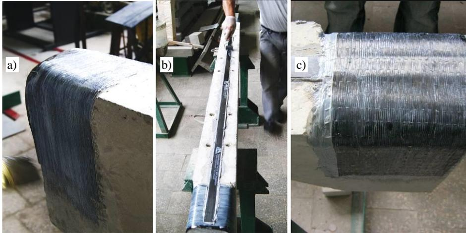
Fig. 2. Applying of first layer of Sika Wrap (a), applying of laminate Sika CarboDur (b), applying of second layer of Sika Wrap (c)
