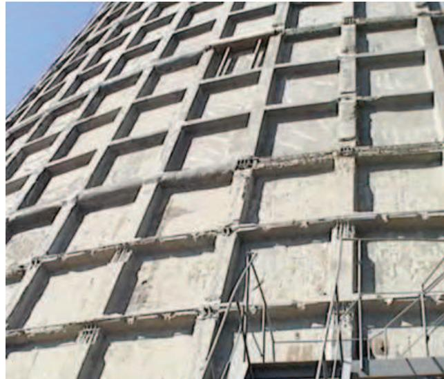
Fig. 6. The outer surface of the shell of the cooling tower during its repair and strengthening of the prestressed armature bars within additional horizontal ribs for stiffness
