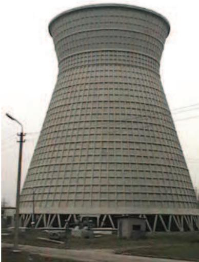
Fig. 5. Prefabricated concrete cooling tower of Darnyts'ka CHP after reconstruction
