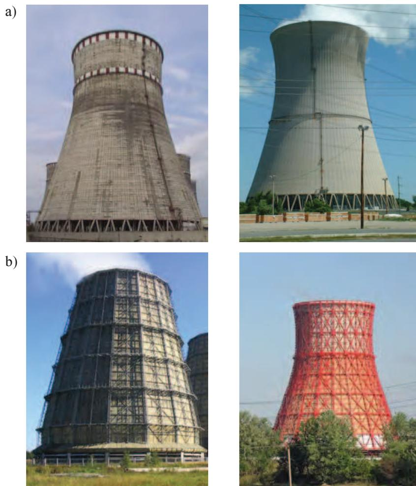
Fig. 1. Cooling towers: a) reinforced concrete, b) metal
