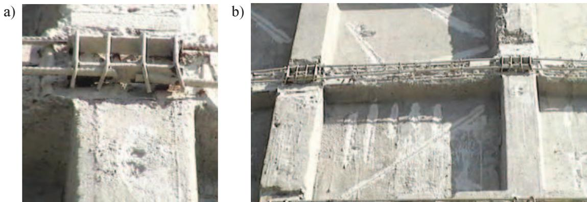
Fig. 4. The process of strengthening performance of horizontal ribs of panels: a) fixation of ring armature on reinforced embedded parts of panels, b) between the embedded parts prestressed reinforcing rods are connected by clamps and fixed to the armature of horizontal ribs
